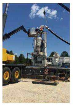
Reverse circulation drilling is a mechanised drilling method that does not require any explosives, thus making it a continuous operation, which in turn achieves higher advance rates.
